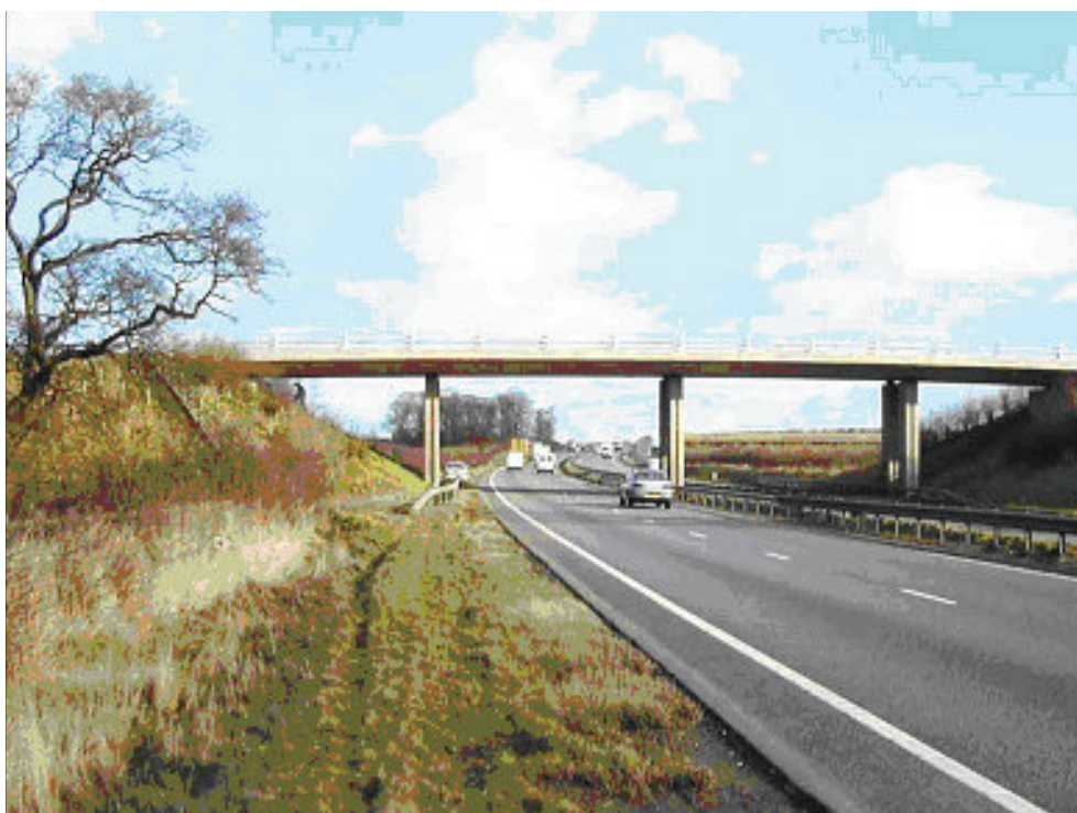
Plate 2-2: Typical Rural All Purpose Dual Carriageway Cross-section
